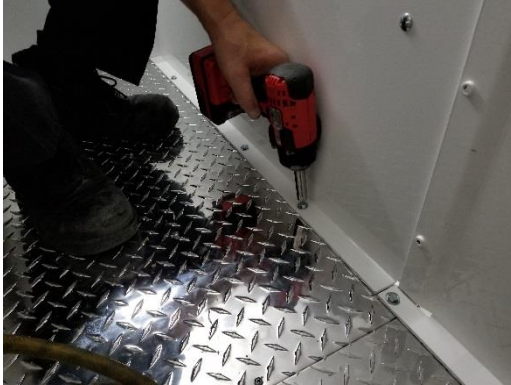
Attach divider to floor with 1/4" x 1.25" #14 lag bolts.
