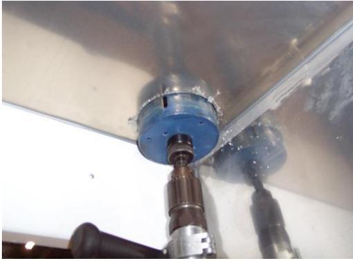
Determine mounting location for camera and mark hole. Be sure to make sure the polycarbonate dome cover fits properly before drilling 4 1/2" hole. Take caution not to drill into any wires.
