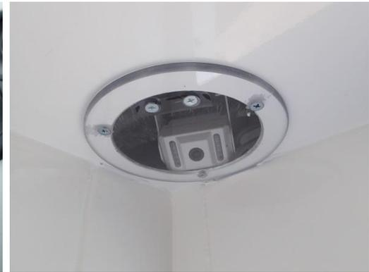
Mark holes on the ceiling and pre-drill with 1/8" drill bit. Reposition camera assembly and mount using #10 x 3/4" Flat head sheet metal screws.
