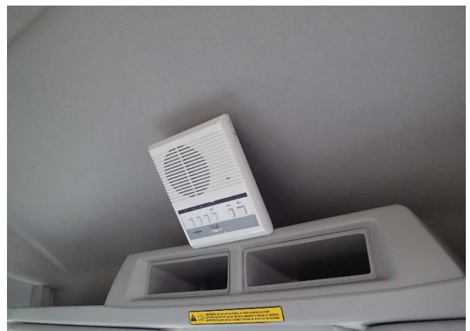
Photo shows master station mounted in alternate location. Bracket modified by installer.
