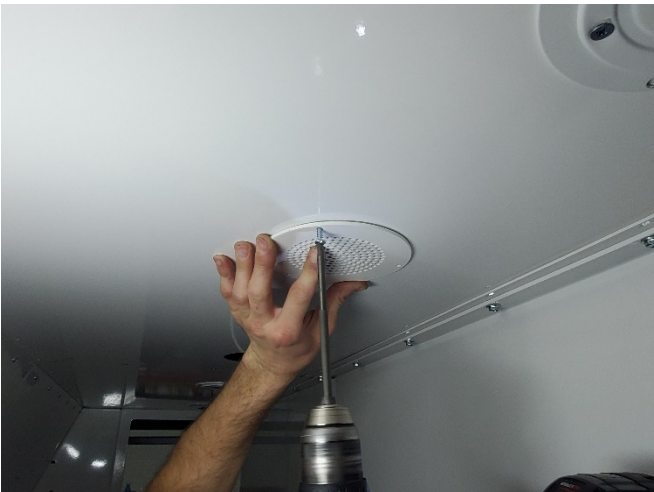
Use supplied #10 Torx screws to attach cover to ceiling of kit.
