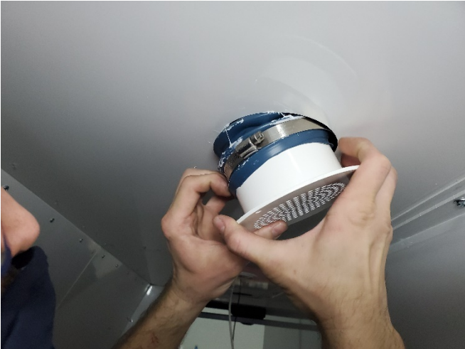
Slide hose clamp over air duct hose and attach hose to vent cover.
