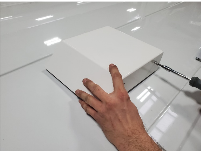
Place cover on lower vent plate and attach together using #10 Torx screws and washers.
