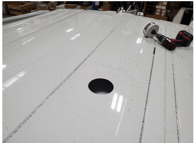
Deburr hole and clean off metal chips.
