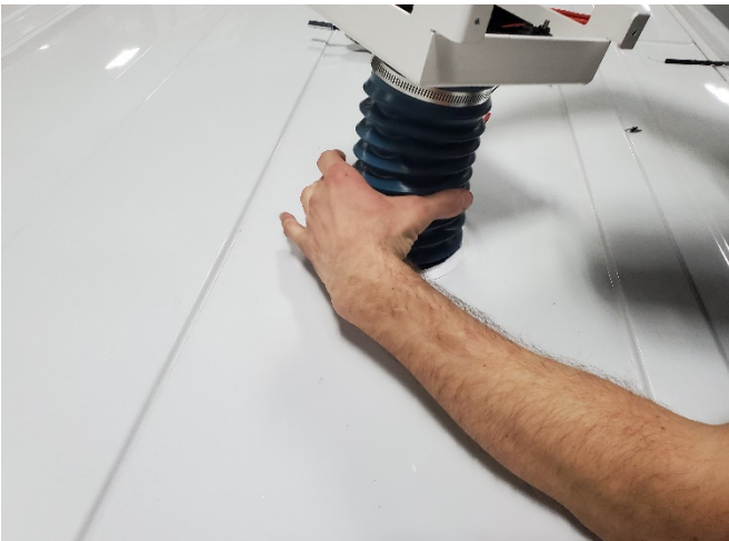
Slide hose through hole in roof. Clamp may need to be inserted at a slight angle to fit through opening in roof.
