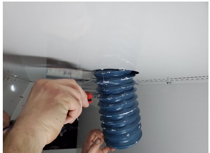
Pull air duct hose through hole in ceiling and cut off excess.
